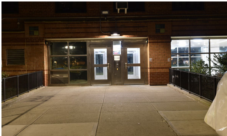
Figure 3. Rear Entry Doors of 439 Beach 54 th Street.
